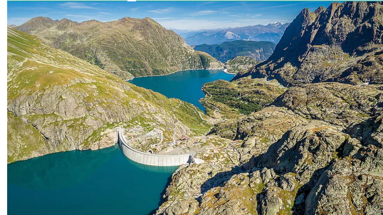
▲ The Nant de Drance hydroelectric power plant uses two reservoirs: the upper Lac du Vieux Emosson, bottom left, and the lower Lac d'Emosson Nant de Drance / Sébastien Moret
